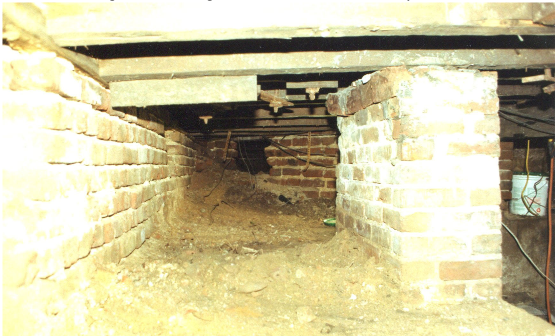
Figure 2-6: West wall of kitchen cellar in 1990.
